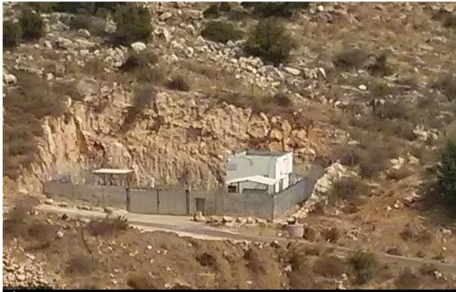
Water and sewage site – north Israel
